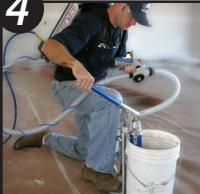
Pump mud from the bucket into the ENFORCER™. The number of pumps required to fill the tank will vary depending on the material viscosity and pump stroke,
