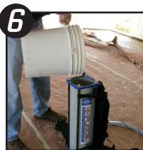
6 Next, fill the tank ¾ full of drywall compound. Insert piston into tank and push down until it is situated on top of the mud. A slight twisting or rocking motion may be necessary to release the air trapped between the piston and the mud.
