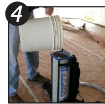
4 Next, fill the tank  $\frac{3}{4}$  full of drywall compound by pouring mixed mud into the top of the tank. Insert piston into tank and push down until it is situated on top of the mud. A slight twisting or rocking motion may be necessary to release the air trapped between the piston and the mud.
